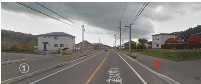
Figure 24. Two sidewalks besides the road
