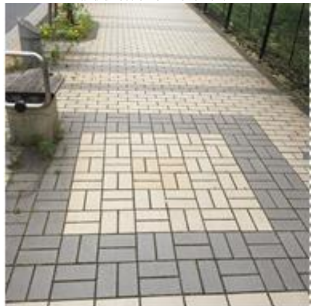
Figure 5. Sidewalk with paver tile
