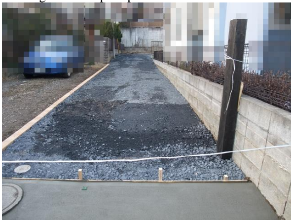
Figure 2. Sidewalk which is under construction
